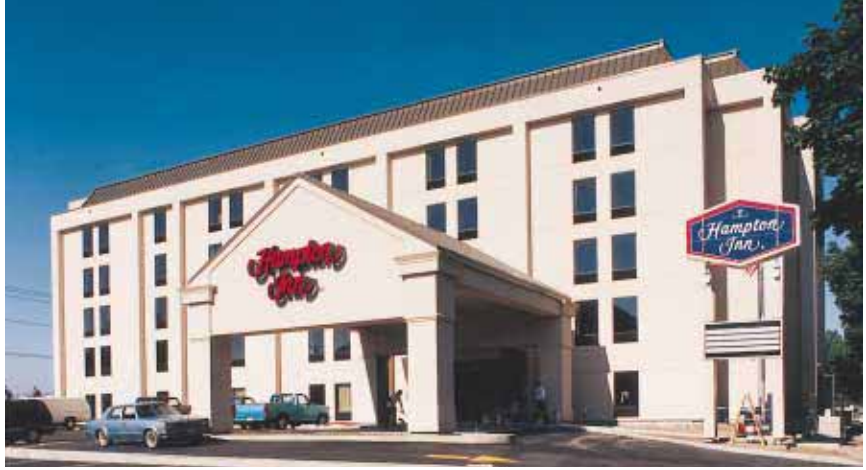
The five-story Hampton Inn in Niagara Falls, N.Y. was constructed during the winter, and the use of precast helped make this schedule possible. The precasters erected the all-precast structure, including load-bearing wall panels, in just five weeks.
