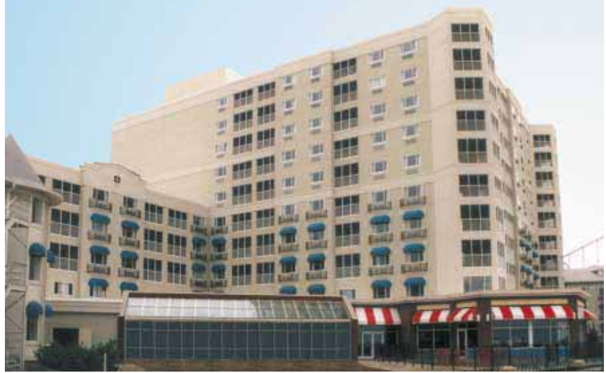
A modular precast structural system, known as the Dyna-Frame system, expedited a difficult construction schedule on the Breakers Tower, an addition to Hotel Breakers at Cedar Point Amusement Park in Sandusky, Ohio. The precast framing system also provided excellent fire resistance, plus sound and thermal insulation. Photo: Davidson, Smith, Certo Architects
