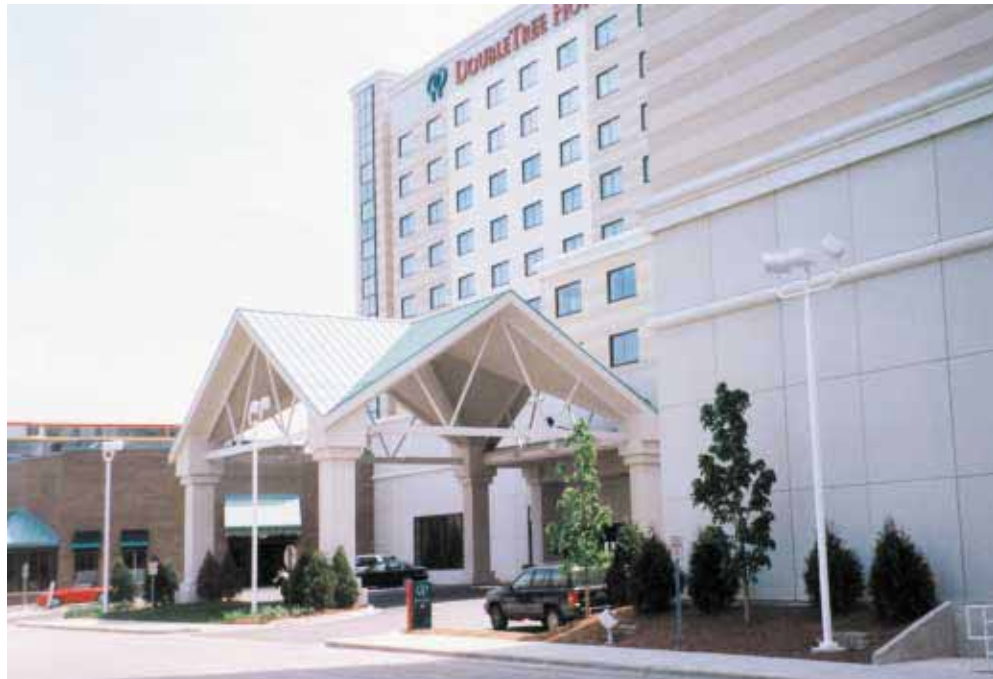
An all-precast building shell was specified for the Double Tree Hotel, Rosemont, Ill., because it is located in proximity to Chicago's O'Hare International Airport and precast is most effective in reducing sound transmission. The finish on the architectural precast wall panels features an exposed sandblasted aggregate on the lower floors of the 10-story building and a smooth finish with horizontal reveals above. Photo: Anthony Rossi
